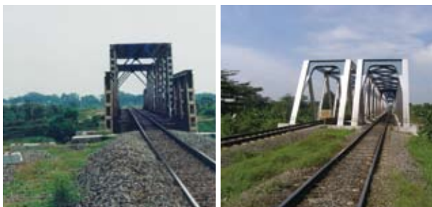
Bridge before project (left). Bridge rehabilitated through this project and separately made to accommodate double tracking (right).
