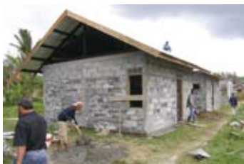
A professor who had studied in Japan applied the techniques he had learned there to develop cement materials that are light and resist water well. This cement contributed to the building of homes during reconstruction.
