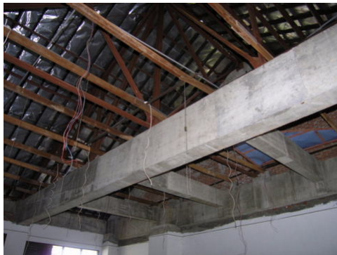
3 rd Floor Ceiling of Engineering Dept. Building
