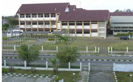
Engineering department building constructed through the project
