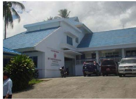
BTS building constructed by the project
