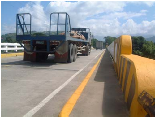
Large Truck Traffic at Indiana Bridge
