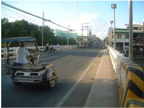
Gumaca Bridge, Rehabilitated in Phase I
