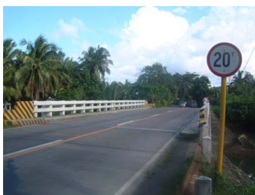
Weight Limit Sign Installed at Talaba Bridge
