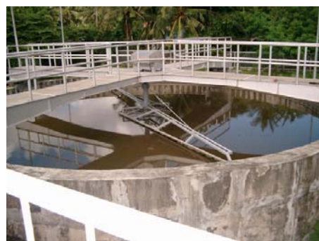
Sewerage treatment plant
