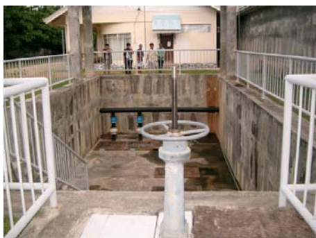
Sewerage treatment plant
