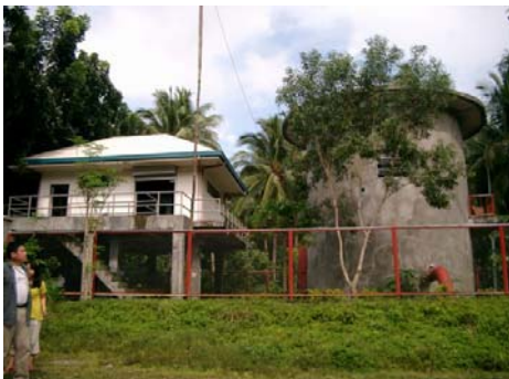
Nabaoy intake plant
