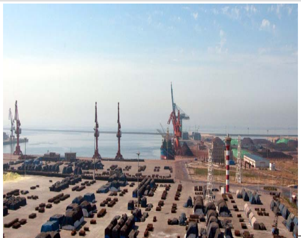
Qinhuangdao Port E and F Berth
