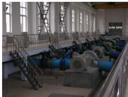
A pumping station developed through this project
