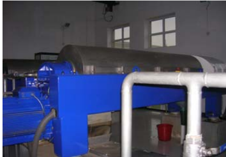
Fig. 3 Facilities to Deal with Sludge
