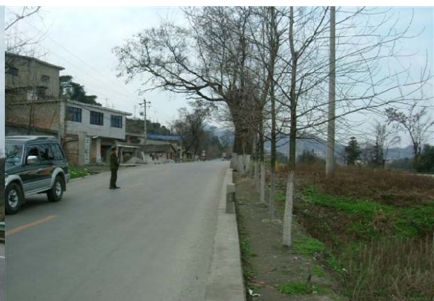
Motorways prior to execution of the project
