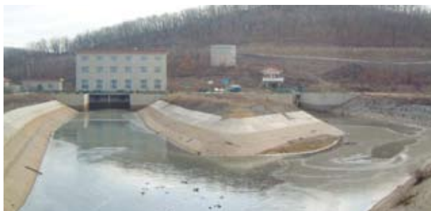
Waterways for power generation (left) and irrigation (right).
