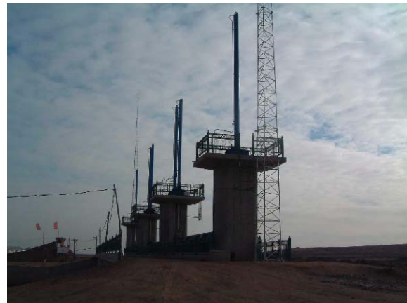
Head works constructed in the Naolihe downstream basin
