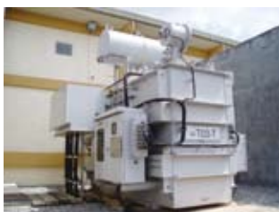
A transformer installed by this project at the Kolonnawa substation
