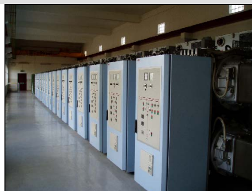
Switching equipment installed through this project
