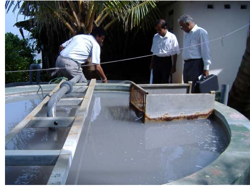
Wastewater treatment plant established
