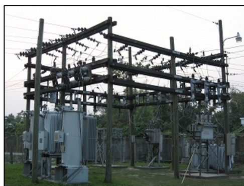
Transformer substation constructed through this project
