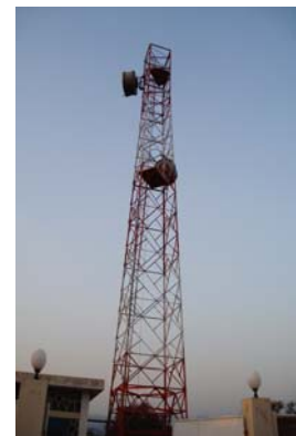
Fig. 2 Microwave System Relay Station
