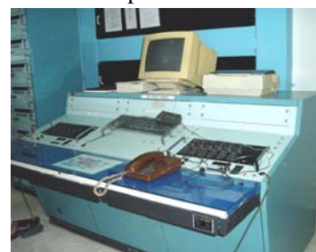
Fig. 6 Maritime Telecommunications Facilities VHF Telephone Console
