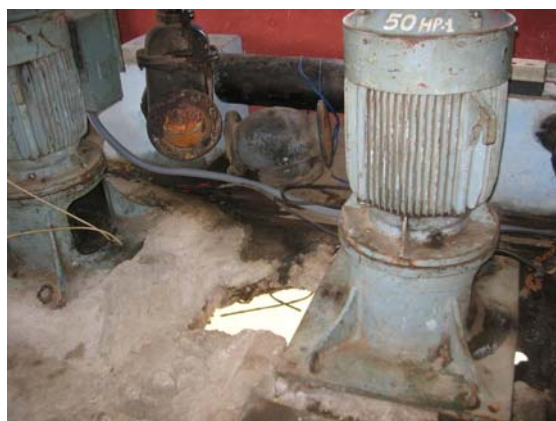
Examples of facilities where proper maintenance is not being kept up (Right) Water utilities in Amritsar: Control panel of deep well pump (Left) Sewerage utilities in Tirupati: Pump motor at sewage treatment plant
