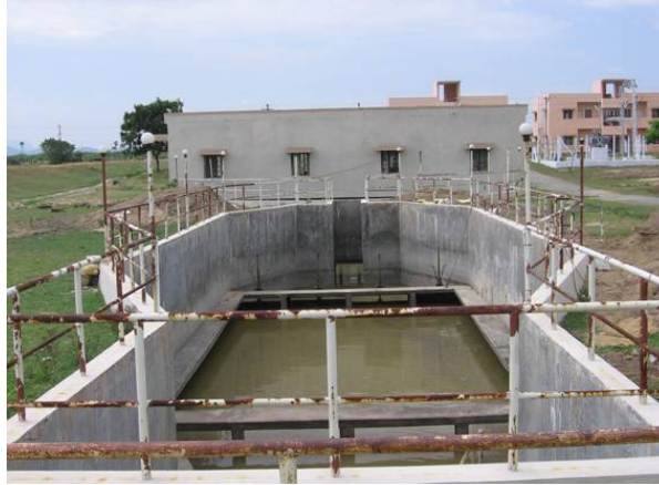
Sewage treatment plant in Tirupati city
