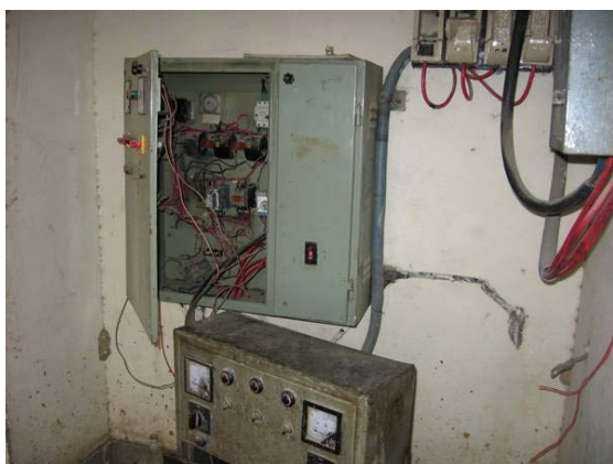
Examples of facilities where proper maintenance is not being kept up (Right) Water utilities in Amritsar: Control panel of deep well pump (Left) Sewerage utilities in Tirupati: Pump motor at sewage treatment plant
