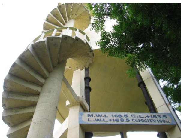
Water distribution tank (Tirupati)
