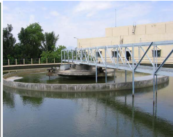
Water purification plant in the city of Tirupati
