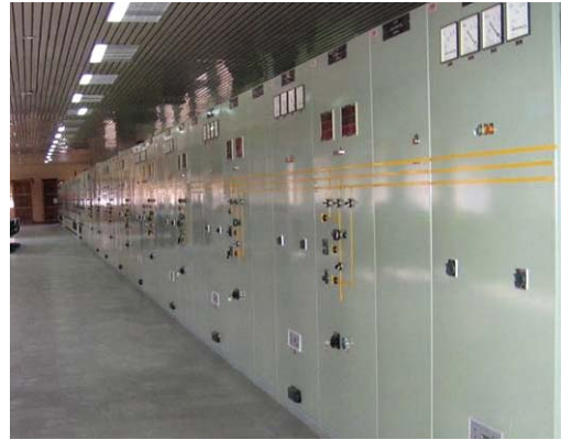
Control panel of the Unnao Transformer
