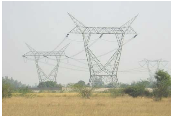
800 kV transmission lines
