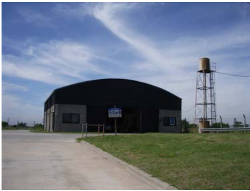
Backwater drainage pump station
