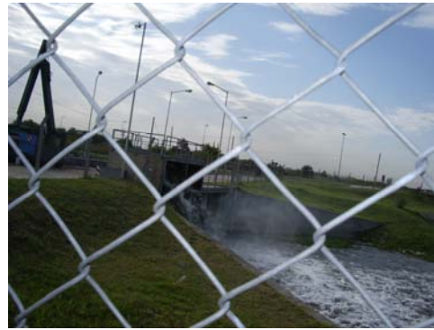
No. 9 (distant view) Draining water
