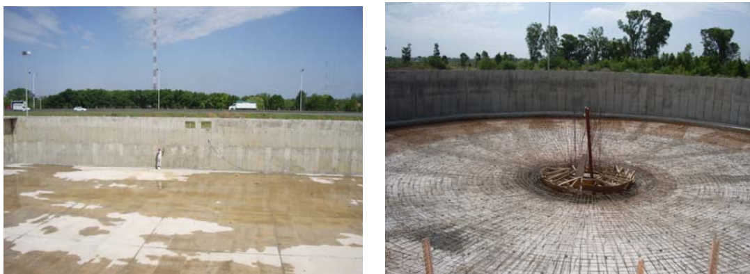
Sewage treatment plants currently under construction (procured through local funds)
