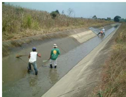
Fig. 3 Cleaning Work Performed on a Canal
