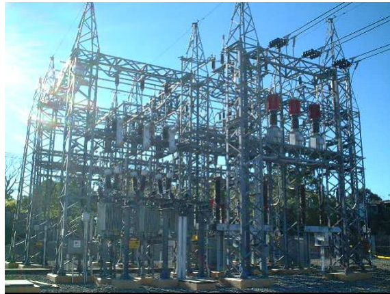
Santo Tomas Substation
