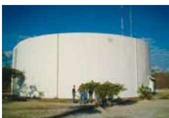
Water storage tank installed by this project
