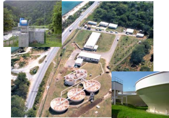
(From left) Water intake system, full view of water purification system, sedimentation tank
