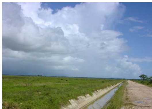
Secondary irrigation channel and farm road
