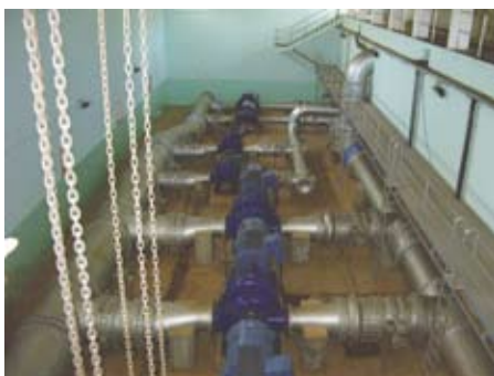
Water drainage system developed by this project at the Lama Pyta supply center
