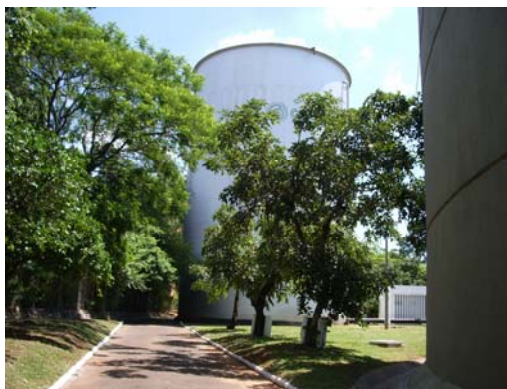
Km 2 elevated tank at a water supply center
