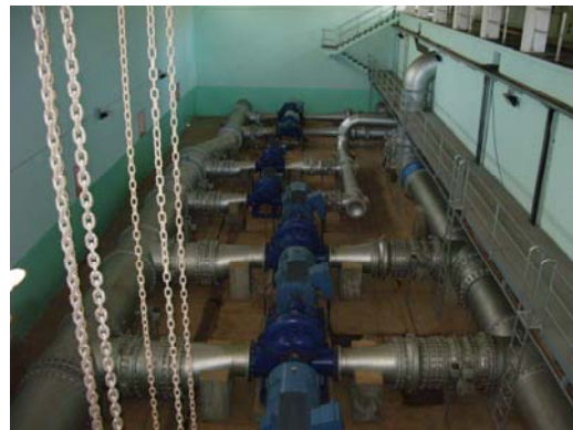
Water distribution pump at the Lama Pyta water supply center
