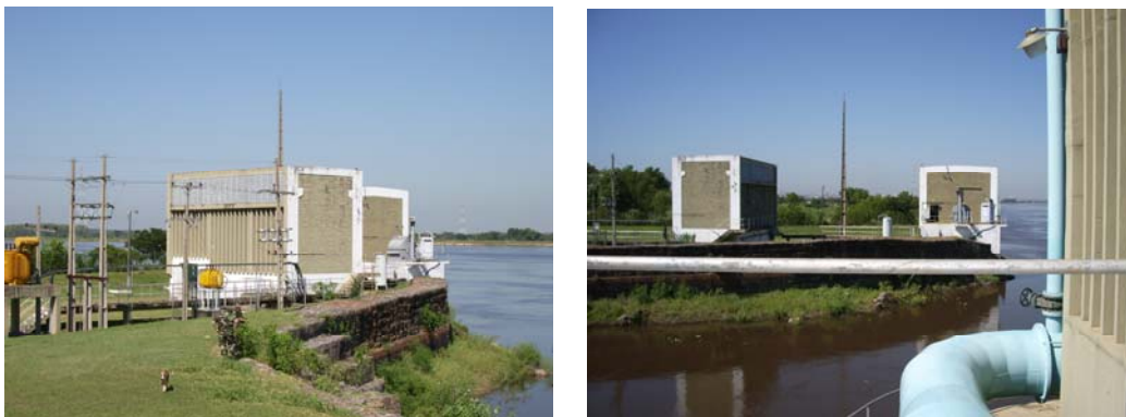
Viñas Cué Water Purification Treatment Plant Facilities
