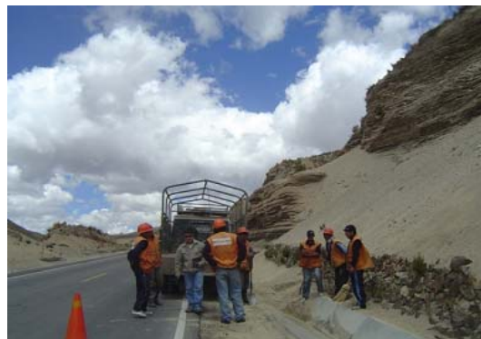
Fig. 9 Routine Maintenance Work
