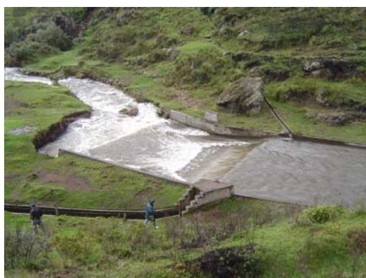
Fig. 1 Irrigation Aqueduct Inlet
