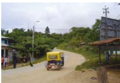
A community road constructed by this project
