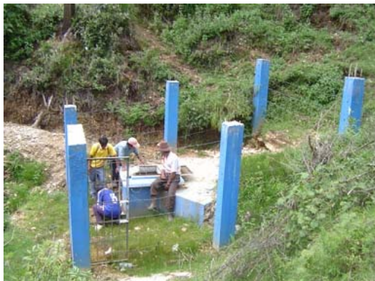
Fig. 14 Potable Water Entrance
