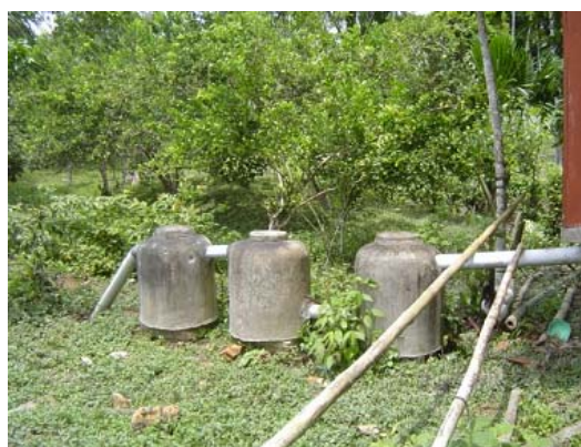
Fig. 7 Latrine Sewage Processing Equipment (Loreto)
