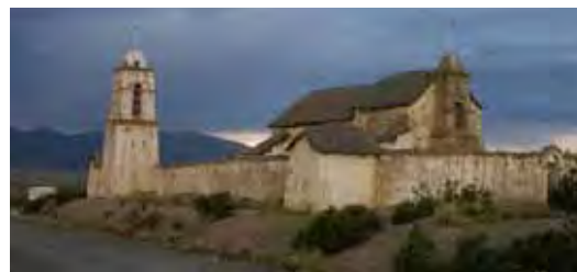
Photo 11. Catholic church where preservation construction was undertaken (Samaja)
