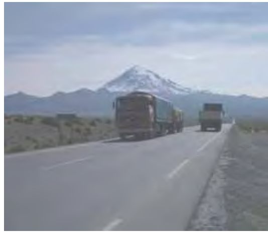
Photo 1: Upgraded road after the project
