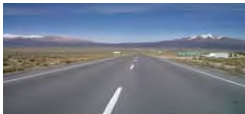
Photo 4. New Upgraded Road (Tambo Quemado environs)
