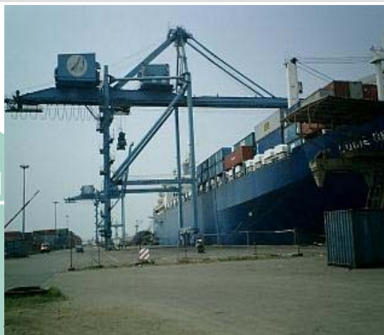
Container crane at Douala Port
