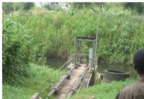
Fig. 3 River Water Intake Facility Volta Region (Hohoe)
