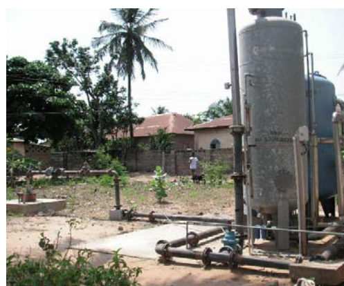
Fig. 1 Water Intake Well Pump and Water Purification Equipment Volta Region (Denu)
