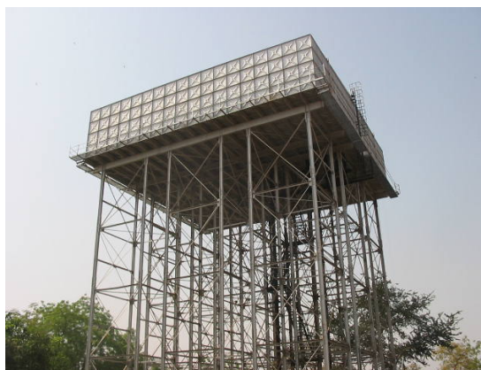
Rehabilitated Water Tower (Tamale)
