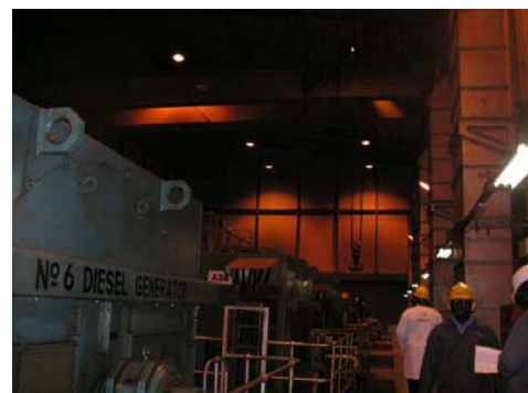
Fig. 1 The six generator units which form the heart of the electric power station
