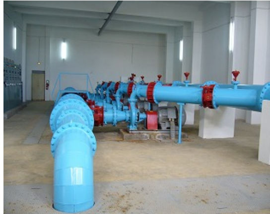
Water supply pump in a water distribution facility
