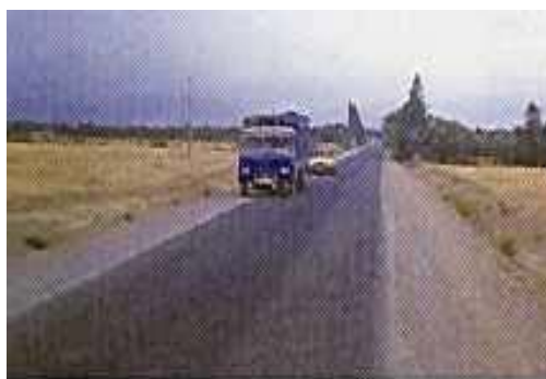
The landscape of the project site after construction works(Courtesy of DRCR)
