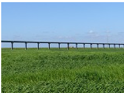
Elevated Water Canal
