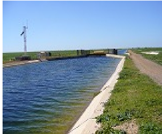
Main Water Canal and Access Road
