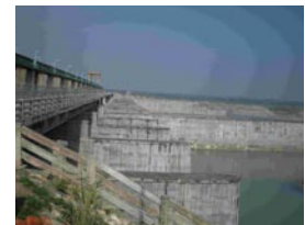
West Yamuna Canal Hydroelectric Project (Downstream of the weir, discharge channels are opened and closed by the gantry crane.)
