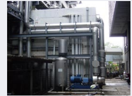
Heat condenser equipment installed at the executing agency.
