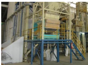
A rice mill plant supported by the project.
