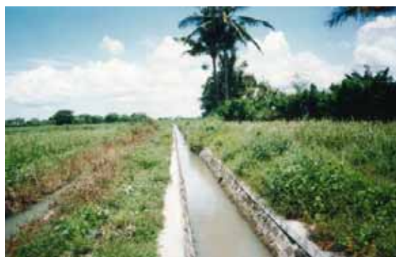
(After Rehabilitation by Project)
