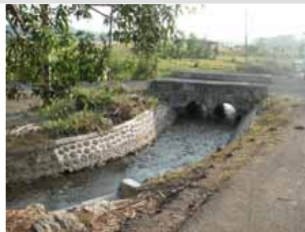
Rehabilitated Lan Lae Secondary Canal South Sulawesi
