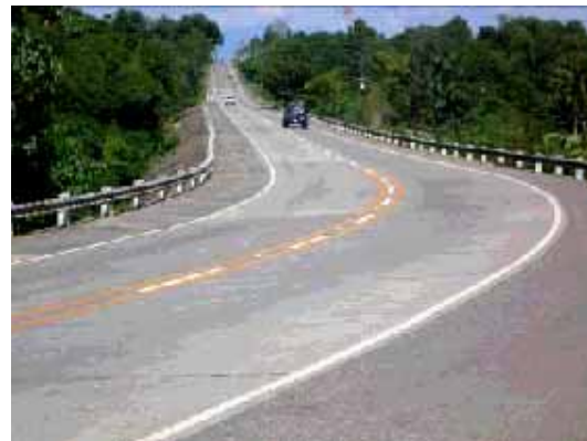
Tumauni-Iguig section of road, part of Phase II
