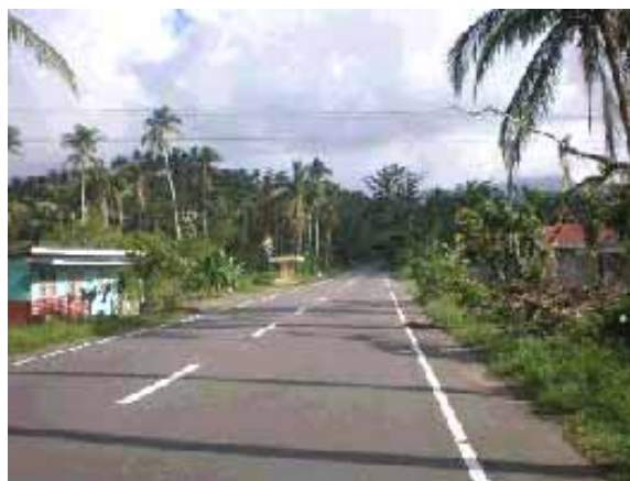
The Daraga-Matnog section of PJFH, a part of Phase II
