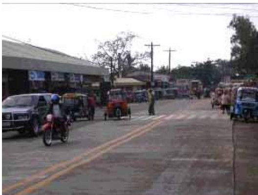
Alcala-Allacapan section of road, part of Phase I
