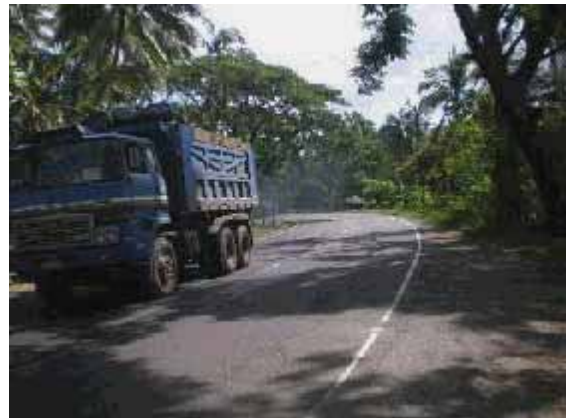
Sipocot-Naga section of road, part of Phase II of the project
