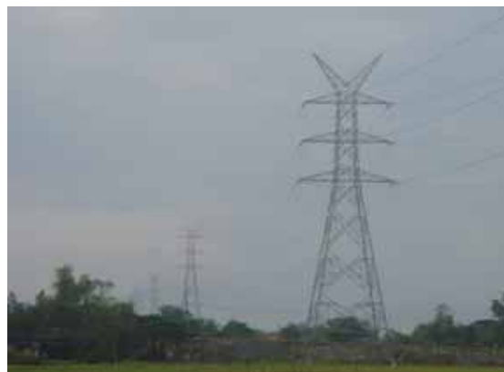
Transmission line to the Casecnan Power Plant
