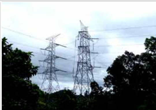
Transmission line connecting the Batangas Power Plant to the existing grid
