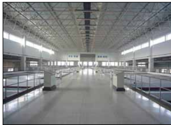
Facilities at Water Purification Plant No. 9 built through Phase III of the project
