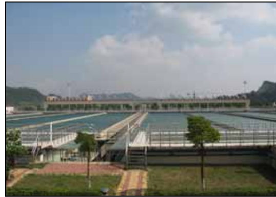
Site photo: Western Suburbs Water Purification Plant
