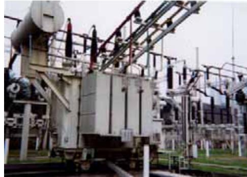
Transformers Installed at the Shaping Transformer Substation
