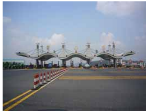
Xiaoshan East Toll Plaza on the Hangzhou-Quzhou Expressway
