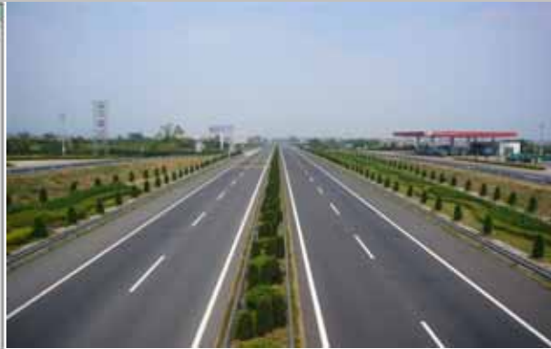
Hangzhou-Quzhou Expressway near the Jinhua Service Area
