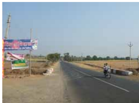
Aurangabad -(Ajanta)- Phulambari segment
