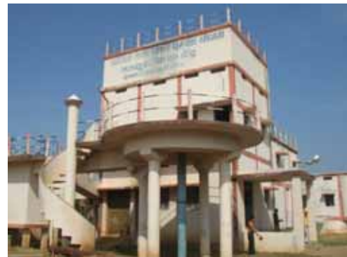
Ajanta Water Treatment Facilities
