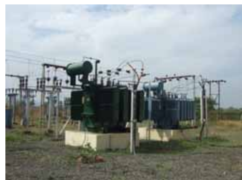
Ellora Power Distribution Facility
