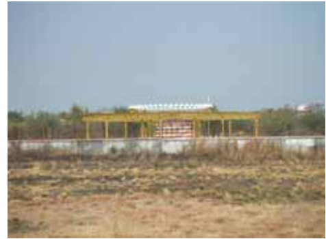
DVOR and DME at Aurangabad Airport
