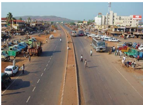
The highway constructed through the project (Chandikhole)
