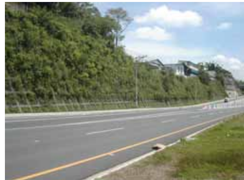
Figure 10: The environmentally-conscious slope introduced in the rehabilitation of the capital's northern trunk road
