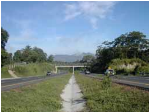
Figure 9: National Highway 1 where a Japanese-style drainage pavement has been applied
