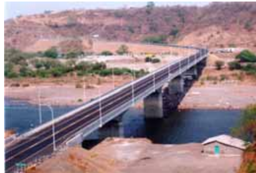
The bridge after the project completion
