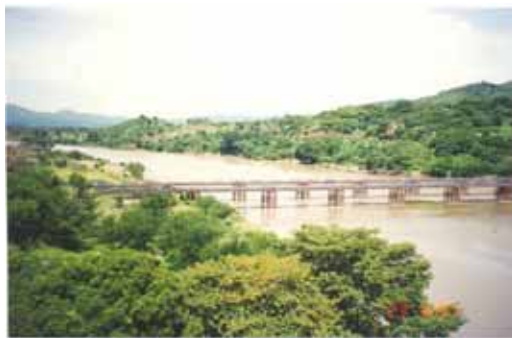
The temporary bridge before the project implementation
