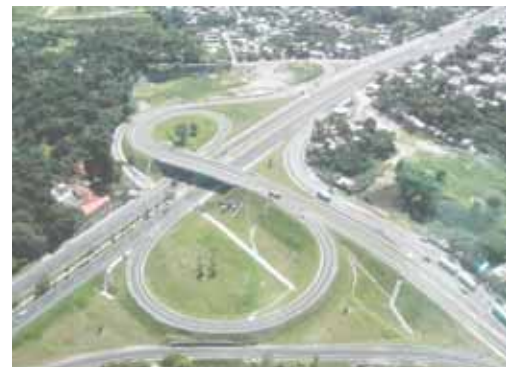
The interchange after project completion
